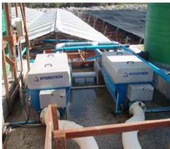
Inlet filters to Abalone farm.
