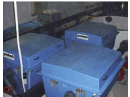
Clean water is collected in a reservoir.
