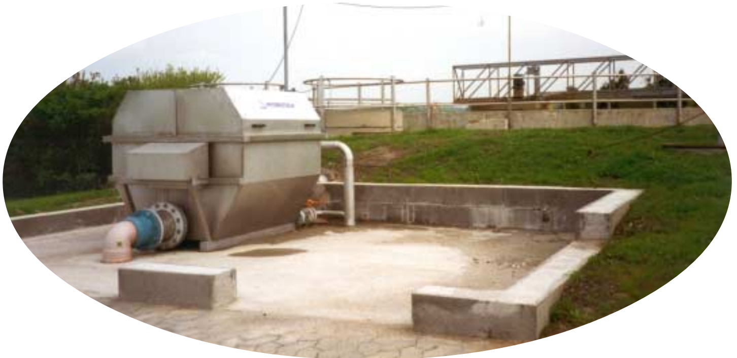
Drumfilter HDF1202-1F as final effluent treatment at Söby WWTP, Denmark
