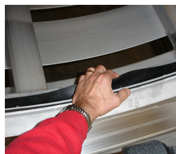
Figure 7.6 Inlet rubber sealing
