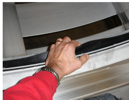
Figure 7.6 Inlet rubber sealing
