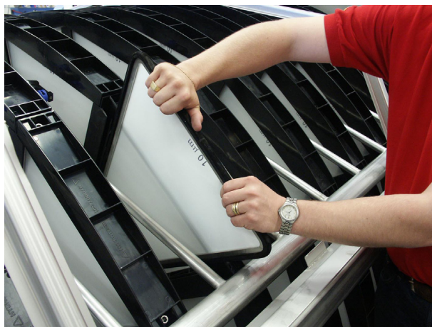
Figure 7.19 The filter panel is pulled out.
