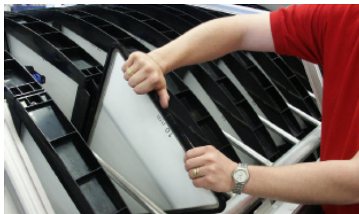
Figure 7.12 The filter panel is pulled out.
