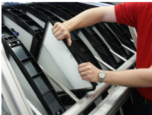
Figur 7.12 Filterpanelen dras ut.
