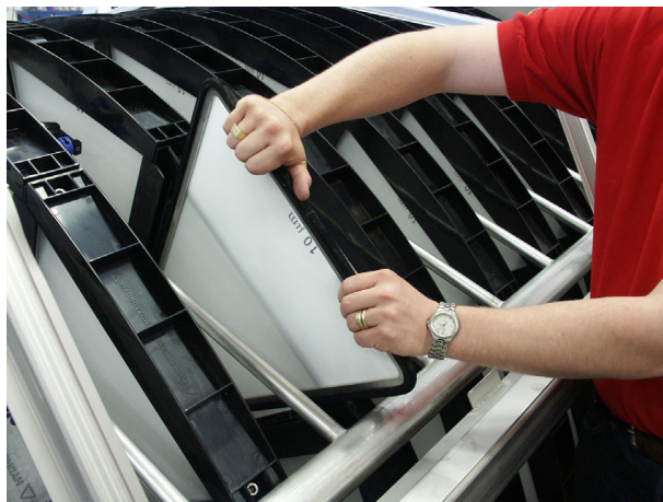
Figur 7.19 Filterpanelen dras ut.
