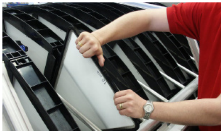
Figure 7.12 The filter panel is pulled out.
