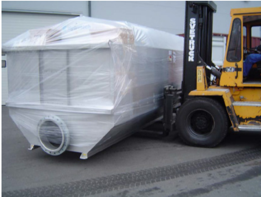
Figure 6, Lifting the filter unit with a fork lift.
